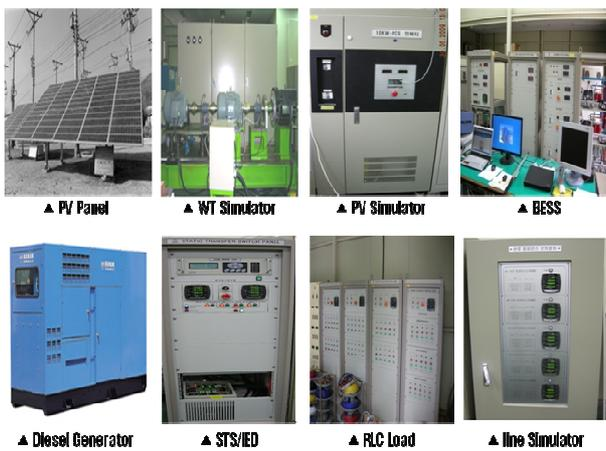
Fig. 8. Feature of the components in microgrid pilot plant.
