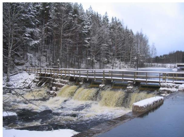
Fig. 2. Part of the dam at the pilot power plant, picture taken 29<sup>th</sup> November 2007. The generator pool is on the right (partially visible). As can be seen, the hydrological situation is such that the inflow is greater than the plant's capacity, and the spillage is high.
