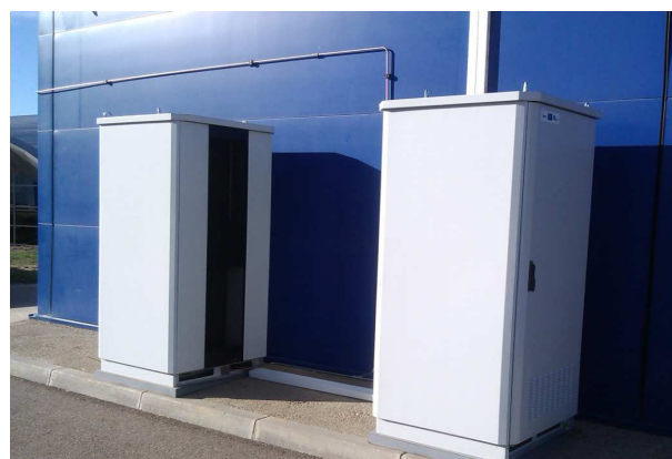
Fig. 8. Fuel cell grid-connected.
