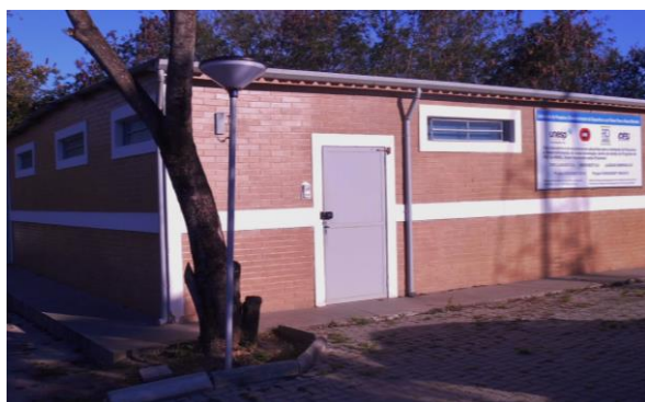
Fig. 2 House built with bricks soil cement.
