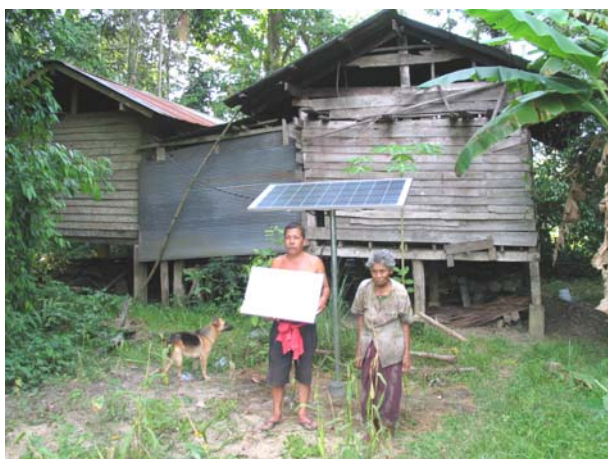
Fig. 5 Typical SHS implementation in Thailand with fixed mounting of PV modules (Photograph: Courtesy Solartron Co., Ltd.)
