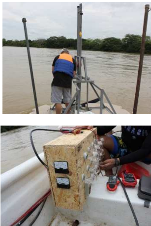
Fig. 8. Installation of the hydrokinetic turbine.
