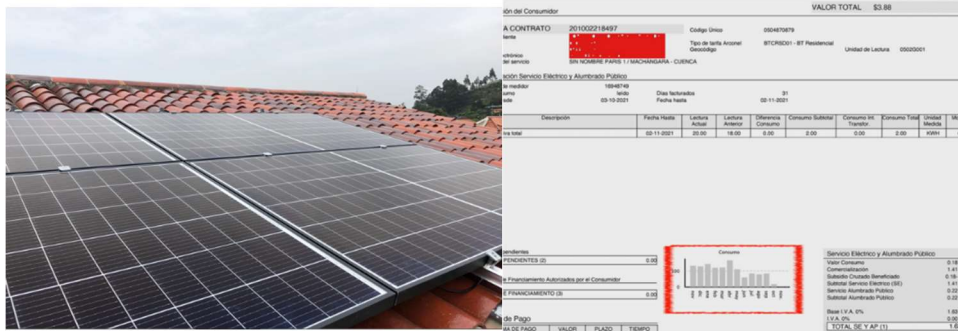
Fig. 5. Single-family dwelling roof with four solar PV plates, and electricity bill with a 2,0 kWh month consumption when starting the bidirectional metering (Source Authors).
