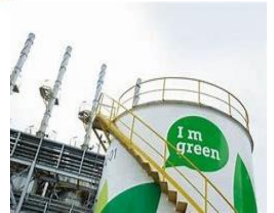
Green Ammonia / eMethanol
