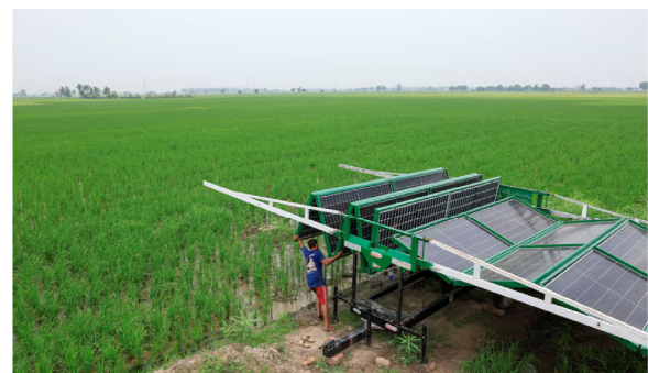
[1/7] A worker installs a folding solar panel unit, to run a tube well, the motorised pump that taps groundwater, in a rice field in Muridke, Sheikhupura District in Punjab province, Pakistan August 12, 2025. REUTERS/Akhil Soomro Purchases Licensing Rights
