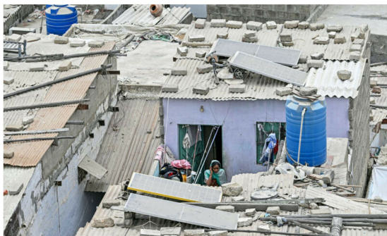
Solar panels are seen installed on rooftops in a slum in Karachi, on June 24, 2025. — AFP
