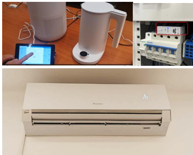
Fig. 4. Water boiler, 3 phase meter for PV metering and air conditioner
