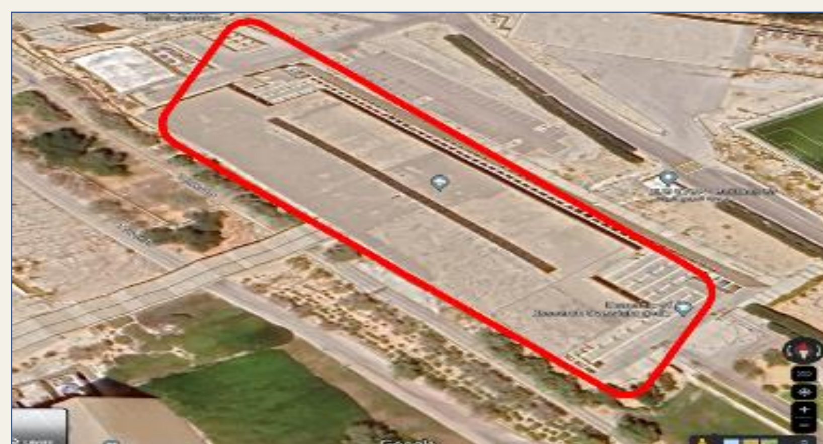
Fig. 3. Area and overview of the selected Academic building.
